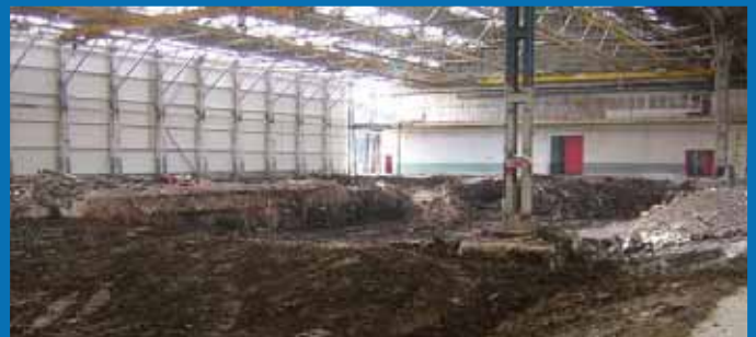
Excavations to remove peat deposit
