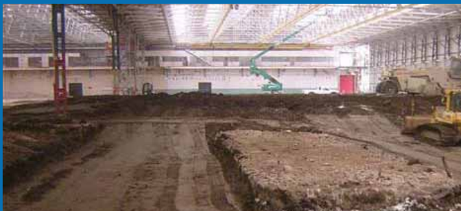
Excavation refilled with lime modified fill (CBR 5%)
