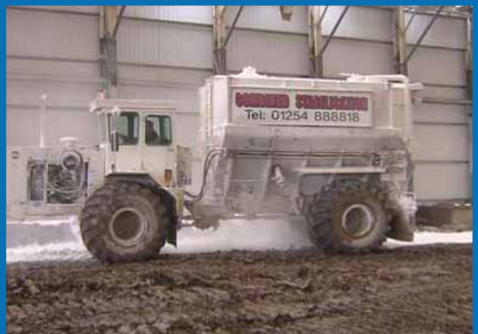
Lime/cement surface layer (CBM 15%), mixed and compacted. Surface sprayed with bitumen emulsion curing membrane
