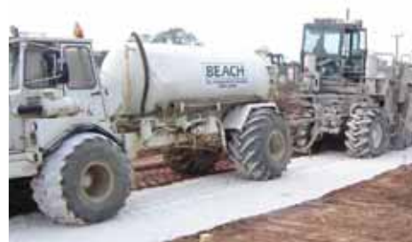
Mixing water into the capping layer
