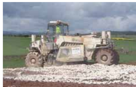
Wirtgen mixing quicklime
